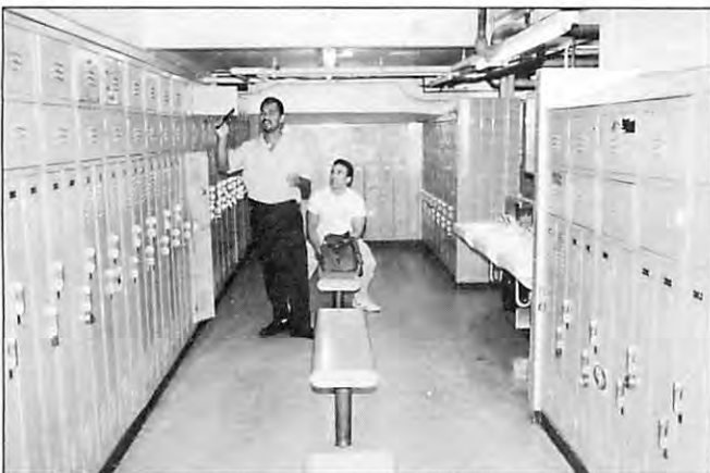
Men and women employees have their own Locker Rooms off the service tunnel by the Purchasing and Store Room areas.
