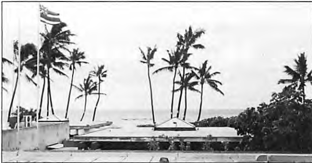
The entire Club was reroofed last fall.
