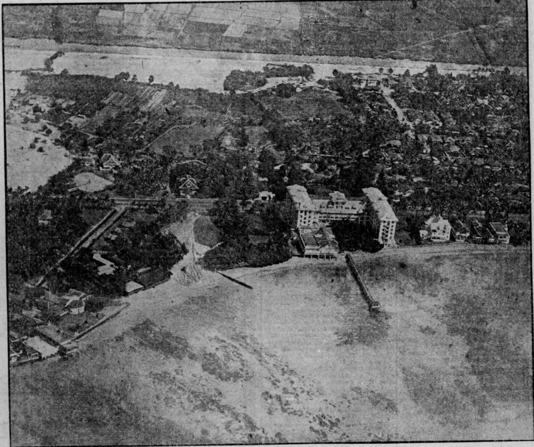
WAIKIKI FROM THE AIR —Land and sea around Moana hotel at Waikiki, as photographed from an airplane. The dark patches in the foreground indicate coral beneath the surface of the water. The Outrigger Canoe Club at the left, and "Heinie's beach" at the right, form, together with the Moana beach and pier, perhaps the world's most famous bathing waters.
