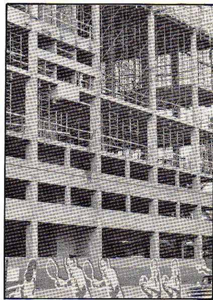
The Honolulu Club is rising on a prime, centrally-located site.
